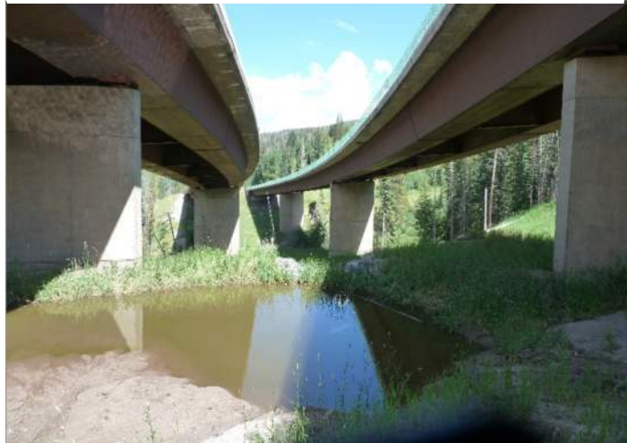
Figure 6. Bridge at MP 185.2 Allows Unimpeded Wildlife Movement Through the Highway Corridor
