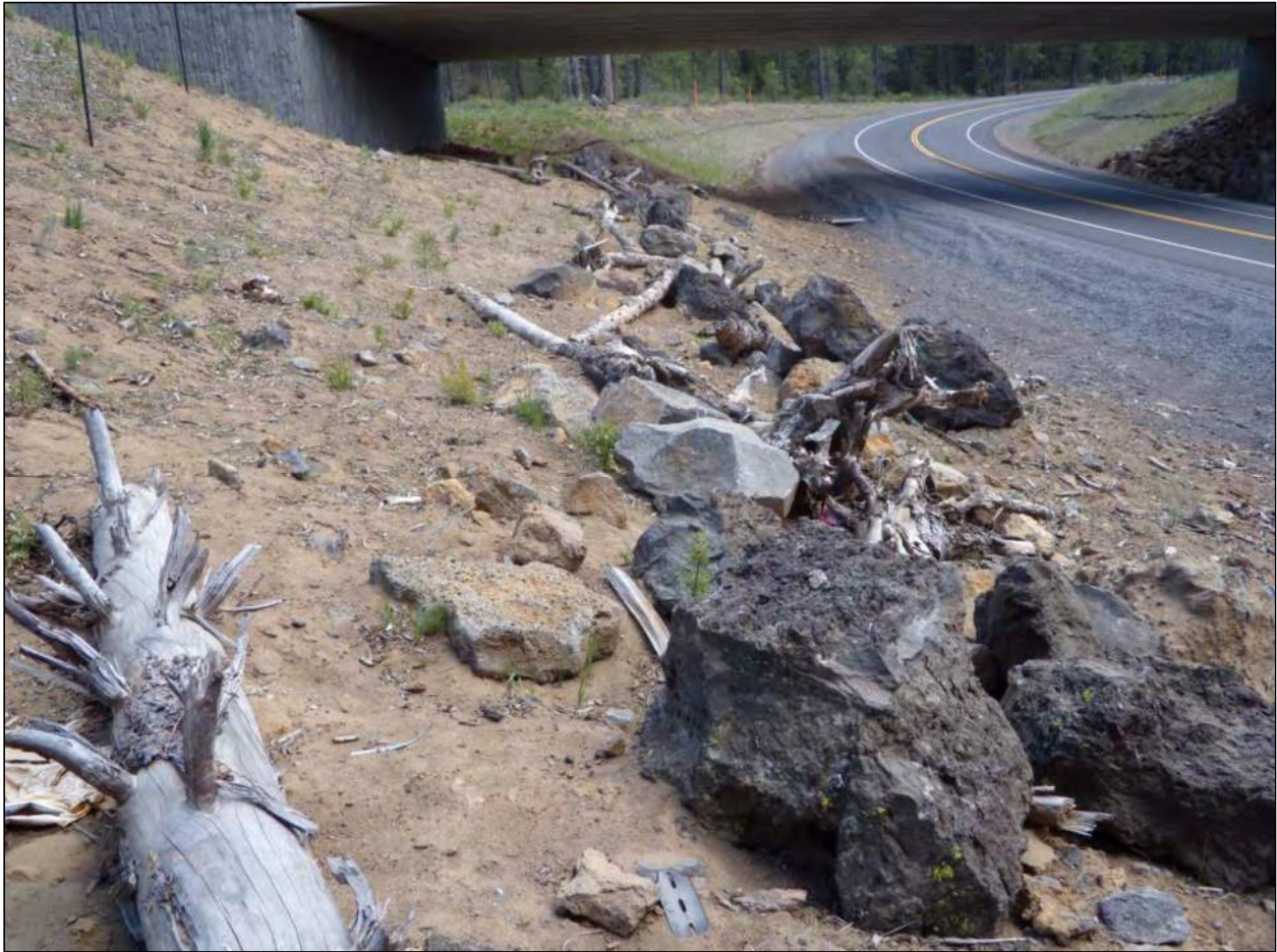
Figure 12. Wildlife lane incorporated into an existing underpass that was originally for vehicle use only. Logs and boulders were added to promote wildlife use.
